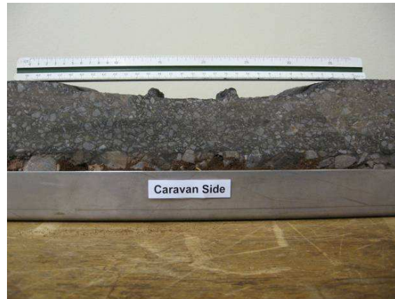
Figure 10. Typical rutting under one tyre in the HMA overlay after HVS testing in the channelised mode using 40 kN and 800 kPa Inflation pressure and 60 °C (n-shape- Dual tyre loading – see Figure 8)
