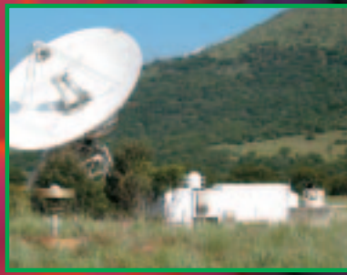
In the foreground is the small Global Positioning System (GPS) basestation antenna at HartRAO. Further back (right) is the Satellite Laser Ranger that measures the paths of satellites, and the big dish of the 26m radio telescope.
